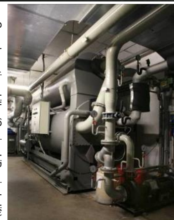
Gas-absorption chiller (Carrier, LIBr, single-lift)
