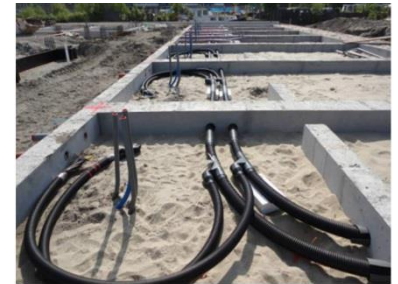
Figure 3: Alkmaar, NL: 6 houses connected to District Heating in 1,5 hrs
