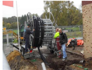
Figure 2: Hengelo, NL: 10 houses connected to the heating grid (2 lines) in 1,5 hrs
