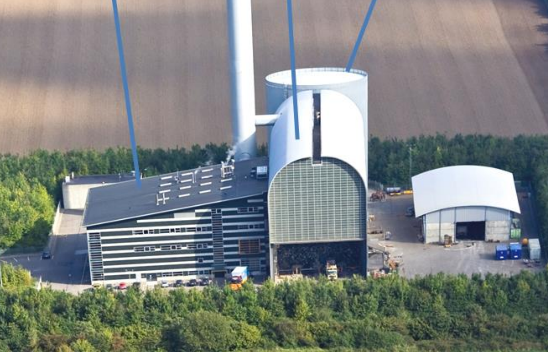
Combined heat and power station – Waste incineration /Gas/steam turbine/Steam
